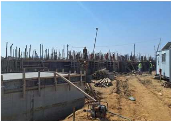
Ground Floor perimeter Beams
