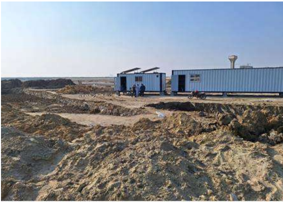
Mobilization on Site
