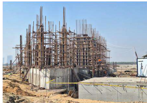
Pouring of Ground Floor to First Floor columns
