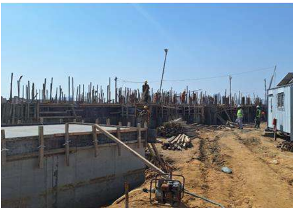
Ground Floor perimeter Beams
