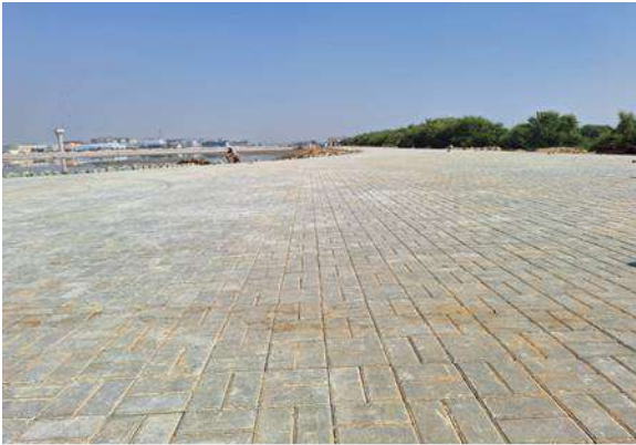
Road works in progress
